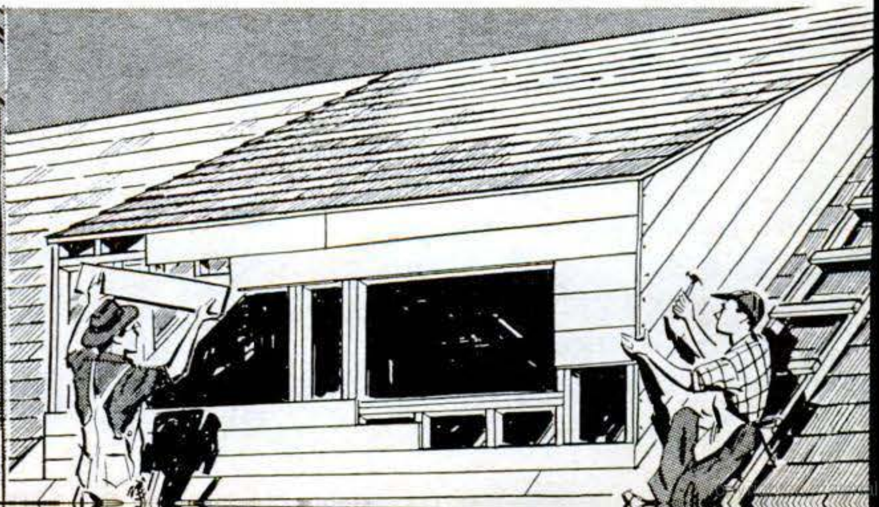
10 SHEATHING is nailed over studs, horizontally on front and diagonally on ends. Use two nails at each stud unless boards are more than 6" wide. Then use three nails.
